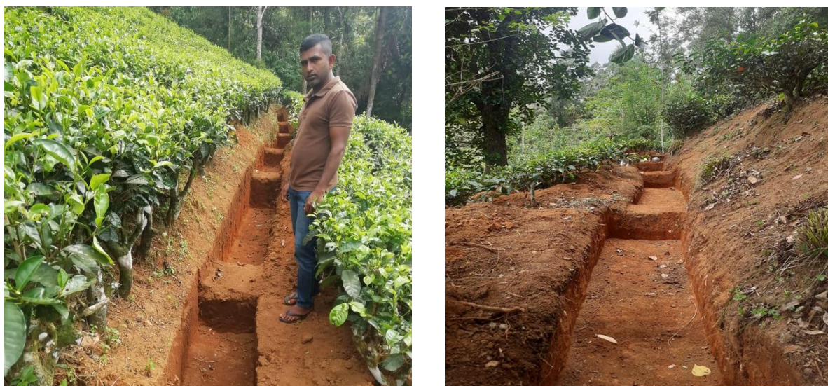
Figure 1 : Program for installation of block drains which is a mechanical soil conservation method in the Ganga Ihala Korale D S division in Kandy District.
