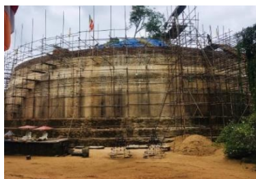
Conservation of Deeghavapi Stupa
