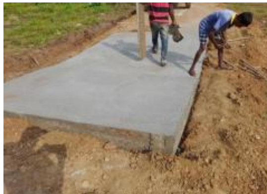
Figure 2-11: Establishment of Concrete Causeways in 2Km Section of the Safari Jeep Track that Runs within Galoya Eco Park
