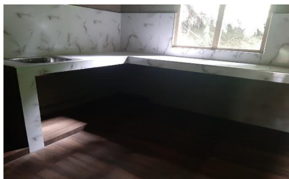
Figure 2-8: Construction of a Kitchen at Makandawa Conservation Centre
