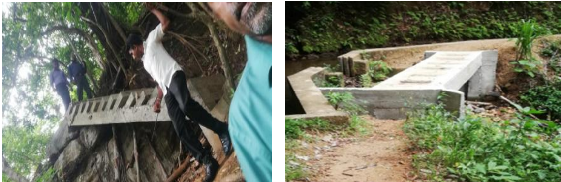
Figure 2-2: Development of Road up to Rathna Ella as an Alternative Road by Constructing Concrete Pillars
