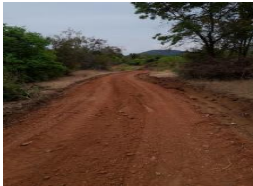
Figure 2-10: Improvement of 2Km Section of the Safari Jeep Track that Runs within Galoya Ecopark
