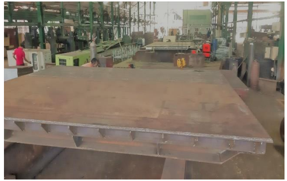
Fabricating gates for Oliyamulla
