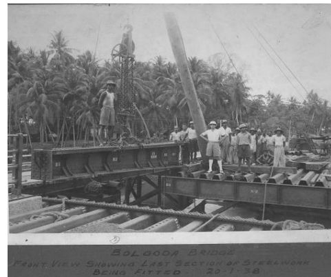
Bolgoda Bridge- Front View
