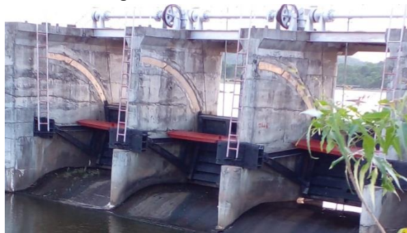
Water control gates at Alikota Ara
