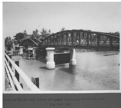
Thoppuwa Bridge 24 October 1938
