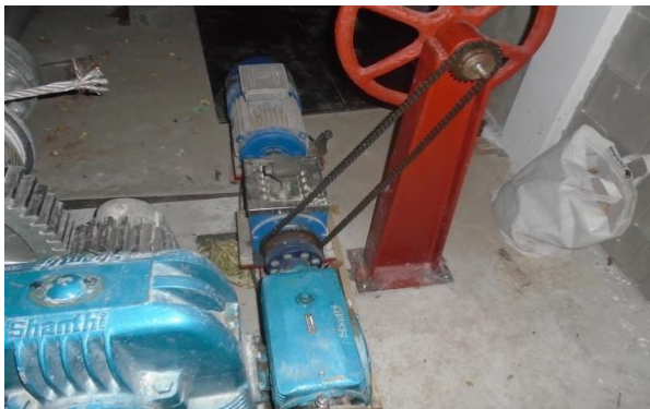
Gate hoisting system of Alikota Ara project
