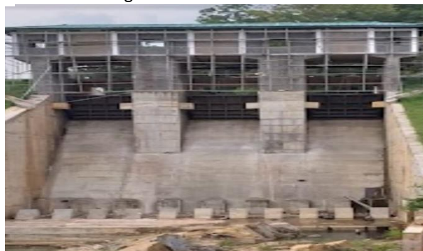
Water control gates at Alikota Ara
