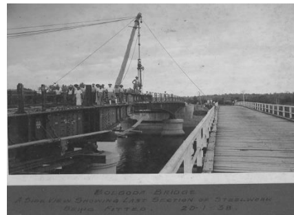
Bolgoda steel bridge –Side view
