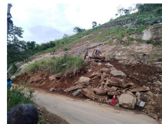
Malapattawa Landslide/RF Site
