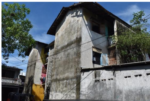
Orugodawatte Majeed Place Housing complex
