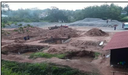
Three storied central armoury building - Panagoda
