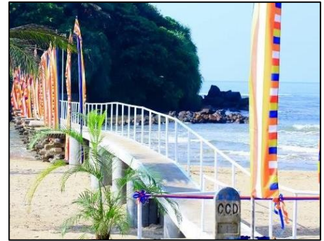
Pedestrian Bridge at Pigeon Island - Matara
