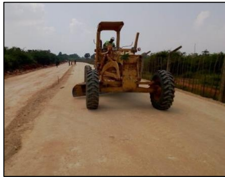
Reconstruct of Myliddy - Kadduwan Road of length
