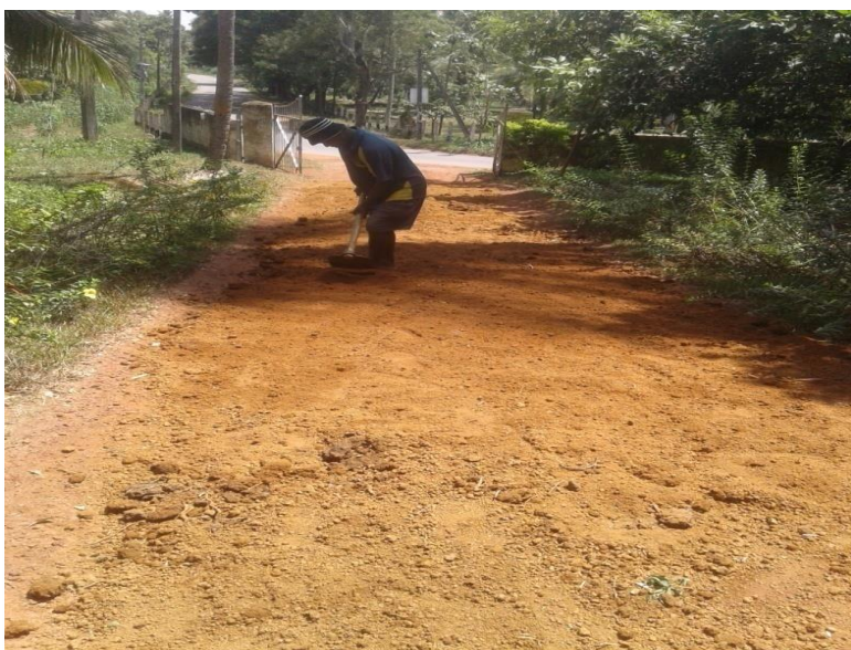
Figure 2.15 In Bopitiya Coconut Model Garden internal roads slanted cross fencing to block wash-off/surface water run-off
