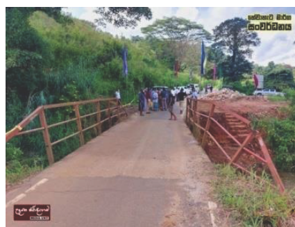
Laying foundation stone for constructing the new bridge of Galaha-Moragallemain road of Delthota Divisional Secretariat with the participation of the Chairman of Pathahewahata Pradheshhiya Sabha and Minister of Parliament Hon.Udayana Kirindigoda
