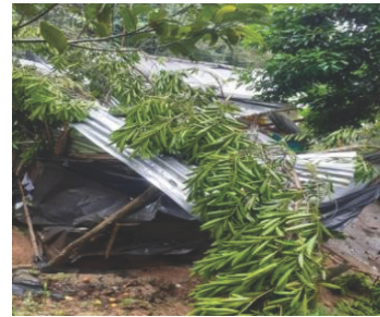
The disaster occurred due to heavy rain in Gopalawatta area of Medawala Harispattuwa Divisional Secretariat
