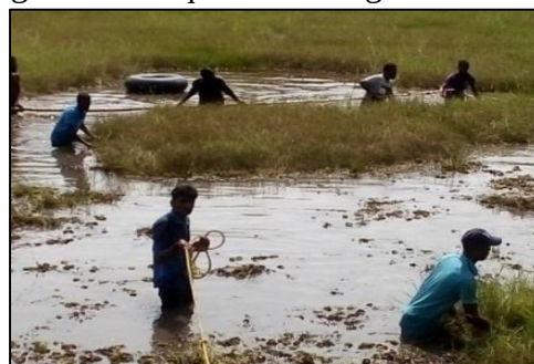
Clearing Small Tanks - Anuraphapura District
