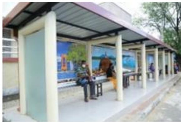
Construction of bus stand in front of Kidney Hospital at 28 th post (Pollonnaruwa M.C.-North Central)
