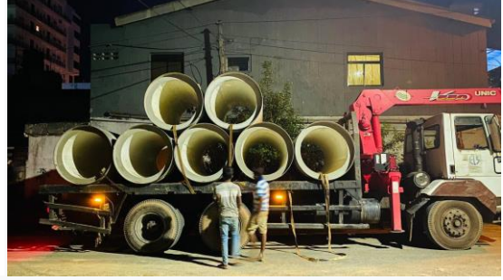
DN 900 RC Jacking pipes were Delivering to the W1 Sites
