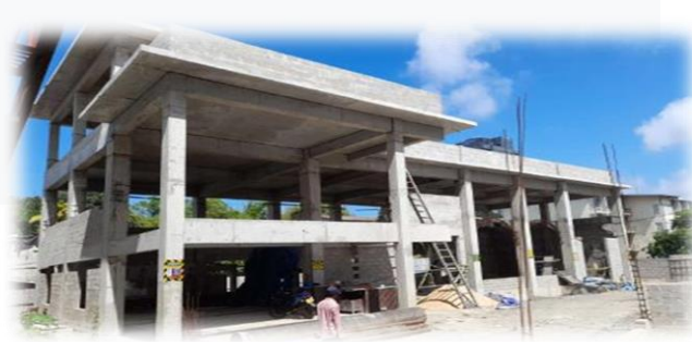
Works at Kalinga Mawatha Pumping Station - Kirulapana
