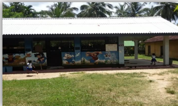
Renovation of Wegama Pre-School (Ridigama P.S. – North West P.)
