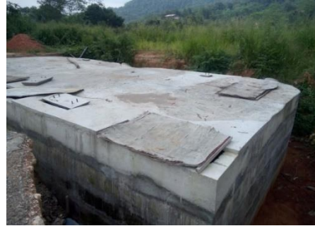
Deraniyagala Bio-Gas Unit
