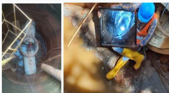
Open cut work is in progress
