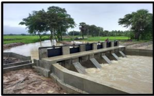
After the development of the Pudumurippu drainage canal in the Karachi local council area of Kilinochchi district
