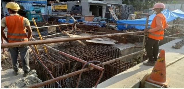
Reinforcement work of column supporting beams CSB 9
