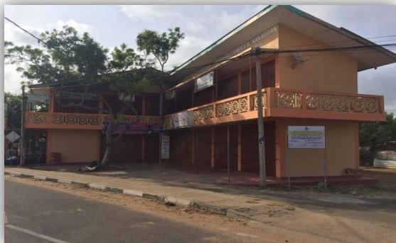
Renovation of Nanattan Shopping Complex (Nanattan P.S.- Northern P.)
