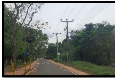
After the rehabilitation of the Puhuleweva Road in Horowpotana Divisional Secretariat of Anuradhapura District
