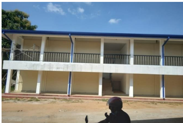
Completion of remaining work new shops complex in Nawagaththegama
