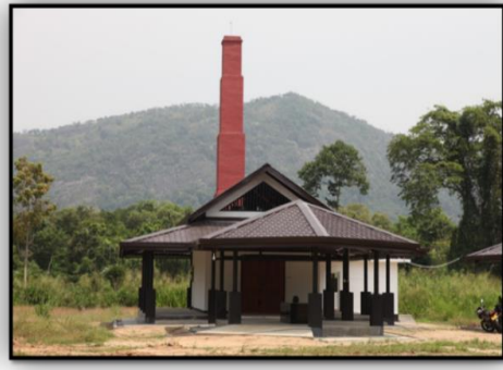
Construction of Madulla Cemetery (Madulla P.S.-Uva Province)
