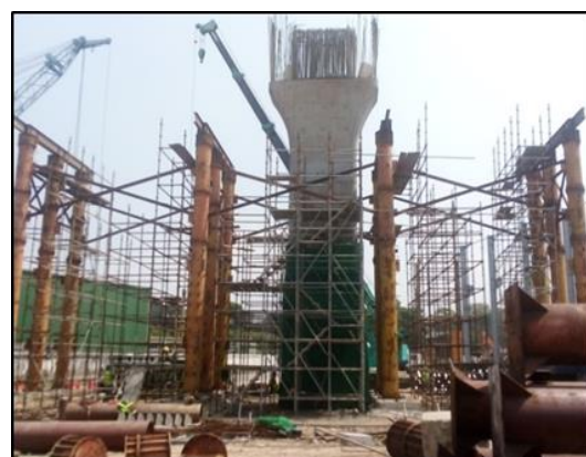
Ongoing constructions at Port Access Road
