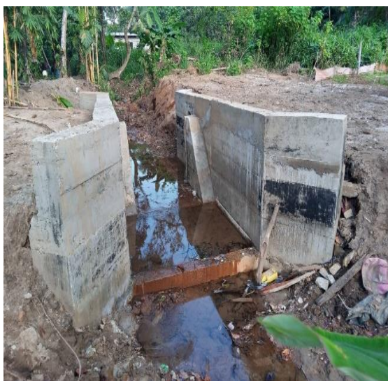
Photo 25 : Renovation of Malwarusha Canal
