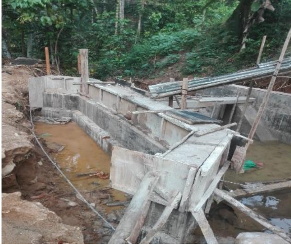
Photo 27 : Construction of Jayavindagama Murutagaha Pela Anicut
