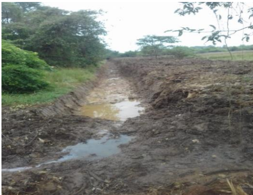
Photo 40 : Ambalaveliya Canal Construction, Puttalam District
