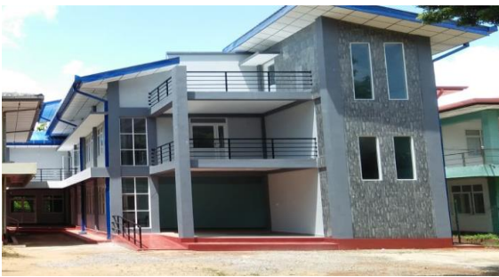
Photo No 30 : Completed Multi-purpose building in Jaffna (Thirunelweli)
