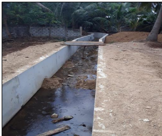
Construction of the sewerage system in the town phase (ii) - Hambantota
