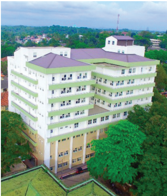
Accident Service, Theatre Complex, I CU and Wards at North Colombo Teaching Hospital - Ragama (Stage III)
