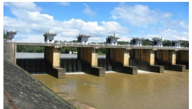
Polgolla Reservoir Capacity: 4.1 million cubic meters
