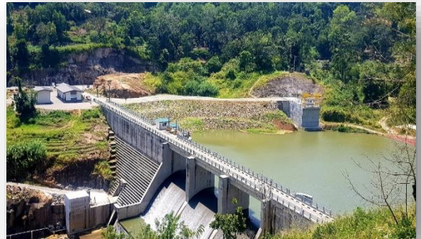
Puhulpola Reservoir Capacity: 0.634 million cubic meters
