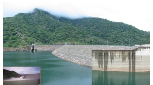
Randenigala Reservoir Capacity: 801 million cubic meters
