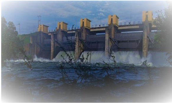
Udawalawa Reservoir Capacity: 268.65 million cubic meters
