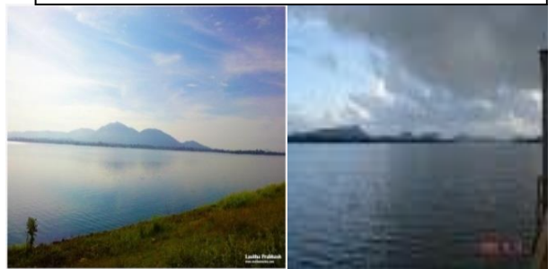
Ulhitiya Rathkinda Reservoir Capacity: 145 million cubic meters
