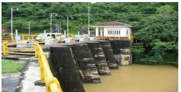
Minipe Reservoir Capacity: 0.12 million cubic meters
