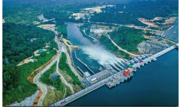
Moragahakanda Reservoir Capacity: 558 million cubic meters
