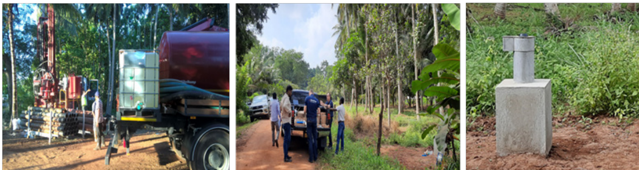
One of the monitoring well during the drilling and the head design and logger installation completed at Rambawa, Malwathu Oya river Basin
