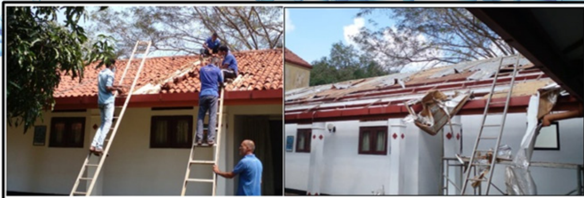
Figure 07: Renovation of roof of Provincial Office – Anuradhapura
