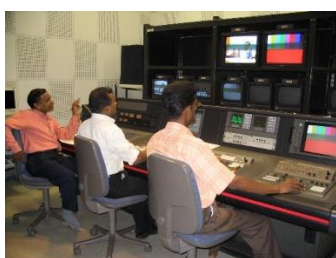
Figure 2a: Control room
