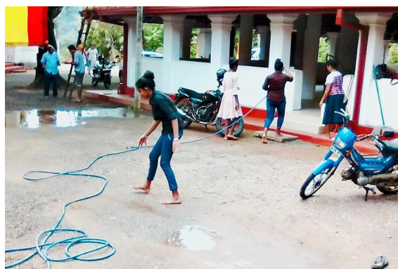
Painting and repairing of Sri Sumanarama temple
