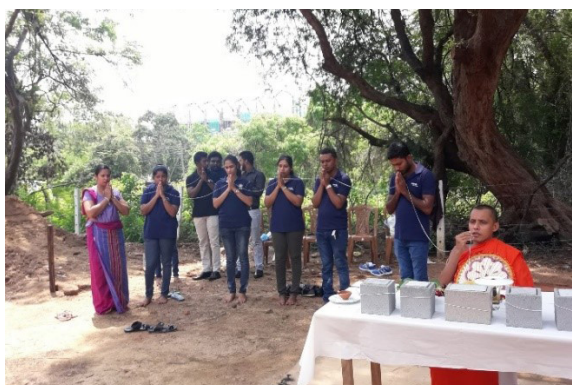
Laying foundation stone for new district office building
