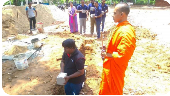
Laying foundation stone for the construction of the new District Office Premises in Polonnaruwa.
