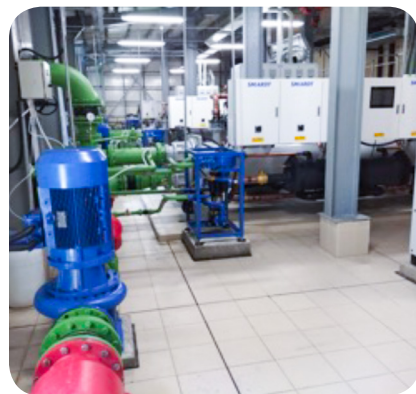
Installation of New Chillers
