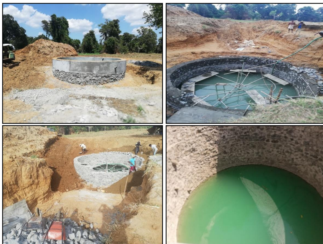
Matale - Wilgamuwa Divisional Secretariat Division construction project for construction of farmer wells (cultivation wells) to minimize damage caused by drought
