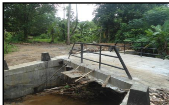
Construction of a small bridge in the place that gets damaged due to floods in Mahara- Bo Maluwa road.
