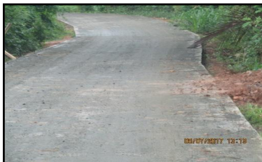
Development of Athuruwela Arambe Galpilla road that was damaged due to the heavy rains in Athuruwela area – Narammala- Kurunegala,
