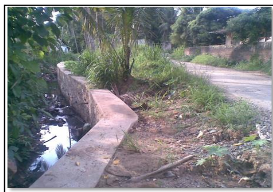
Developing canals to reduce landslides - Udunuwara
