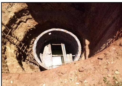
Constructing wells to mitigate effects of drought – Mullaitivu District
