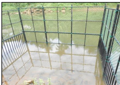
Safe bathing places – Matara district (Minimizing hazards caused by Crocodiles)
