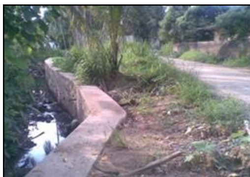
Developing drainage systems to minimize landslides - Udunuwara
