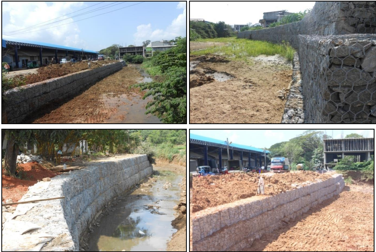
Mitigating floods in Dambulla
