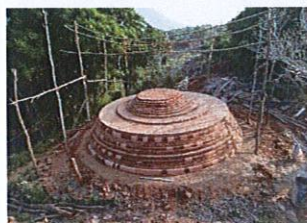
Kaduruwewa Archeological site – Conservation of Terrace and Courtyard
