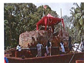
Conservation of Stupa – Eppawala Pothgul Viharaya
