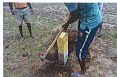
Fixing boundary posts at Ampara
