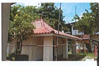
Sankhapitiya Viharaya Kaduvela- Conservation of Image House
