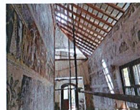
Conservation of the roof of Thelikada Sunandaramaya
