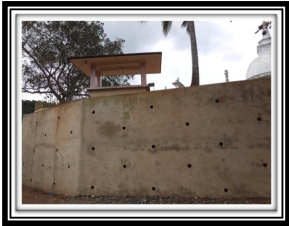
Construction of protective side wall of Sri Sasanalankara ancient temple in Udagama
