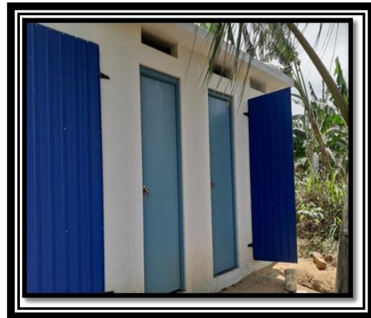
Construction of toilet system at Sri Wanawasee Yogasramya in Sewanagala divisional secretariat
