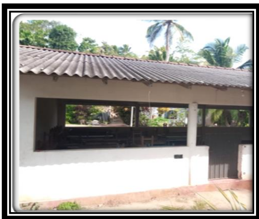
Construction of Sri Wimala Dhamma School Building in Madampagama Divisional Secretariat
