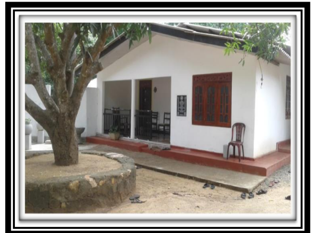
Reconstruction of the monastery of the Sri Dhamma Pranitarama Temple at Kiriibbanwewa, Welioya, Mullaitivu
