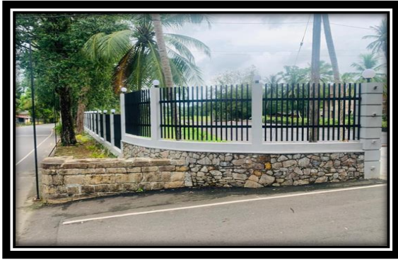
Construction of the security fence of the Olaboduwa Raja Maha Viharaya
