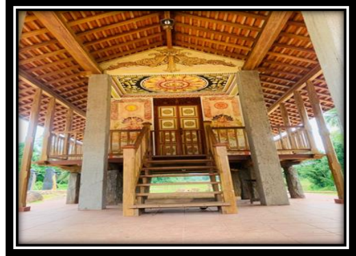
Renovation of the Tampita Vihara of the Olaboduwa Raja Maha Viharaya
