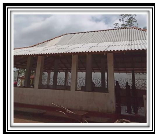
Renovation of the roof of the Dharmashala of the Sri Asokarama Temple in Udawelivititalawa
