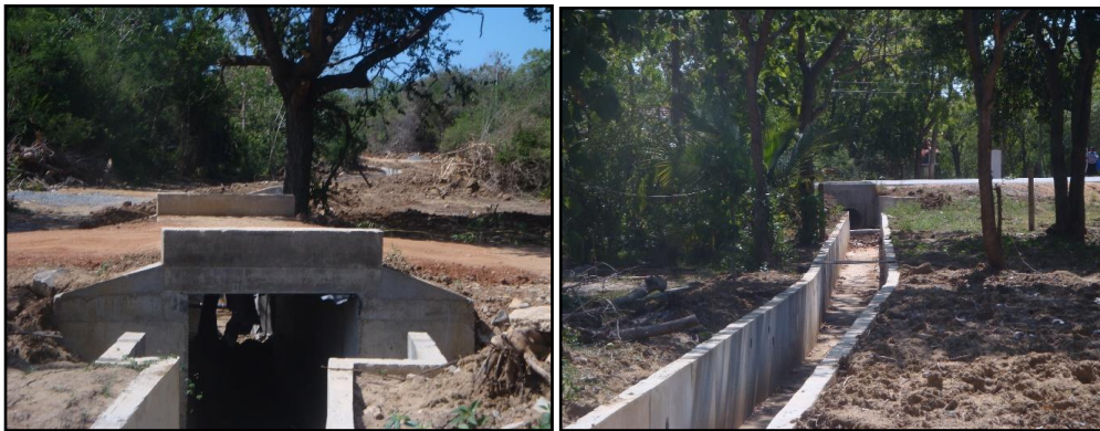
Construction of gutters to remove rain water in Hambantota, Uhapitigama
