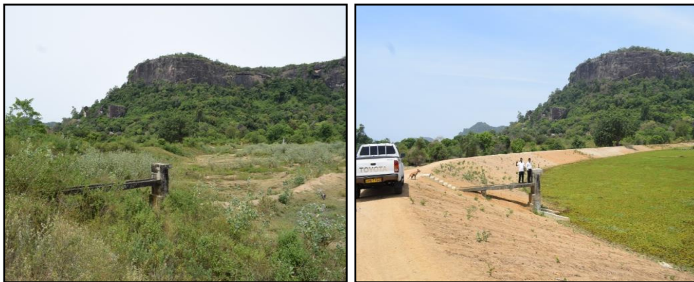
Construction of the bund of the Saddatissa tank in Polonnaruwa - Kandegama
