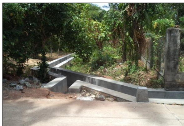
Reconstruction of the water drainage system from Uthuru Mirissan Kotuwa, Nawa Kotuwa up to Kulama wewa- Puttalam
