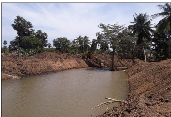
Construction of the Mahawewa Vaan Ela- Trincomalee
