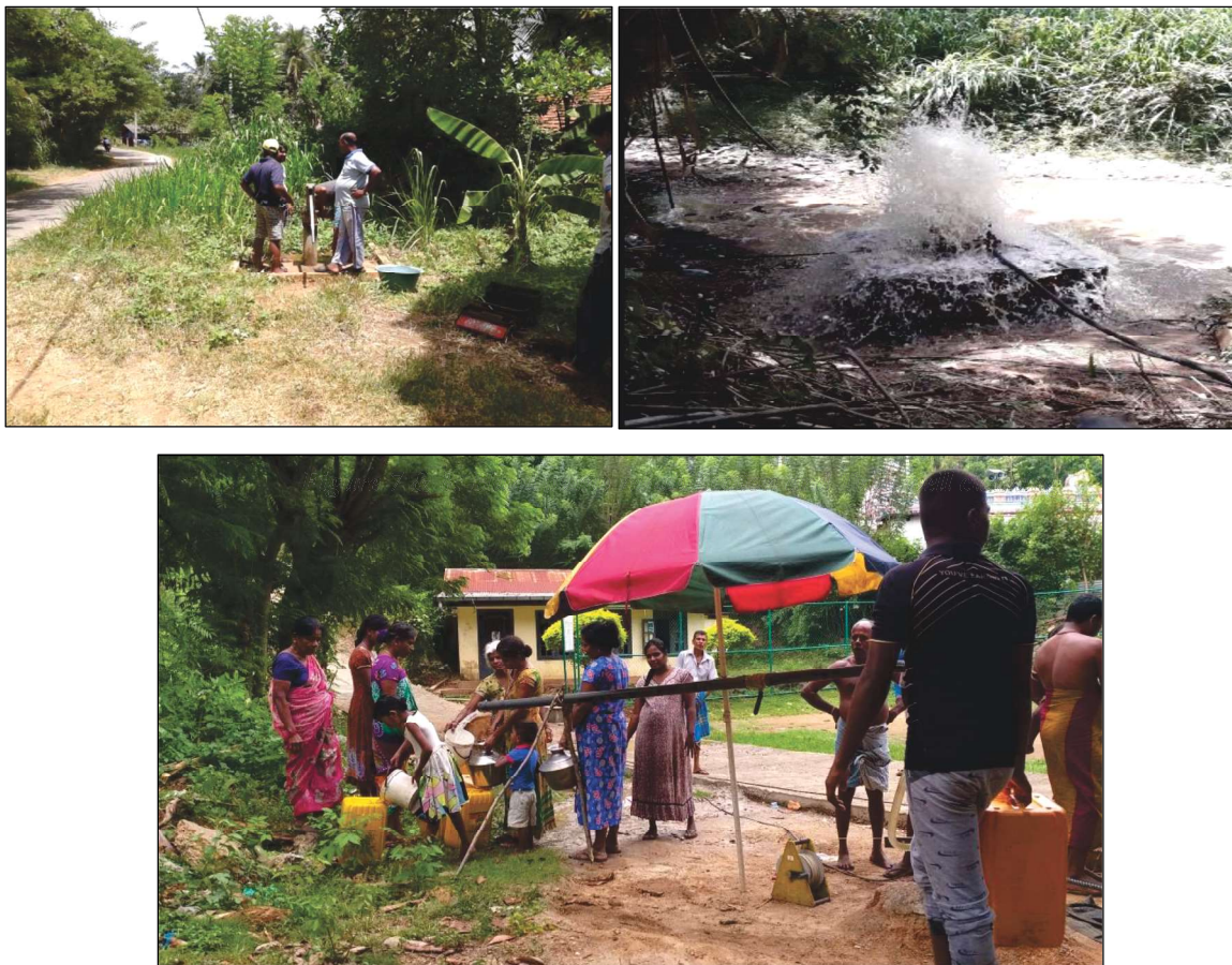
Figure 9: Rural community use water from constructed Tube well
