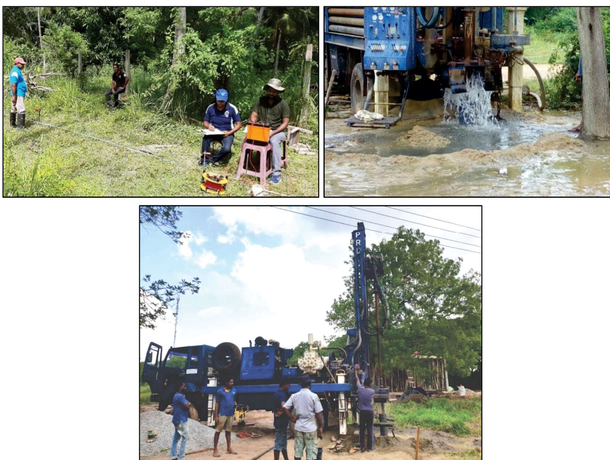
Figure 5 & 6: Carried out Hydrogeological Survey and Construction of Tube Wells.
