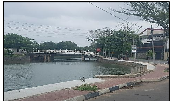
Improvement work on the Gabion Wall along the Heen Ela
