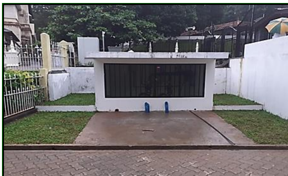
Pump house for sprinkler system
