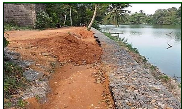
Embankment filling of the lake
