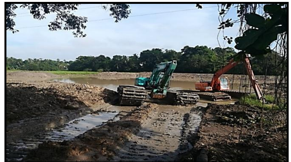
Construction of Proposed Wetland Park 'Siyatha' at Gampaha
