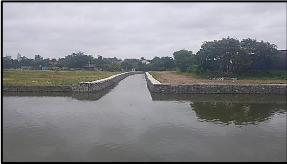
Construction of Gabion Wall at Heen Ela
