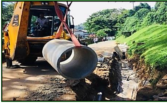
Hume pipe culvert construction
