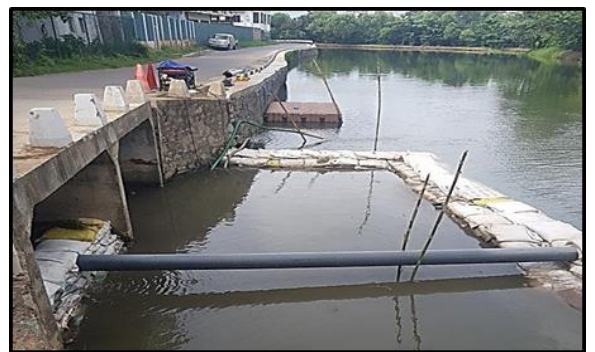
Widening of Culvert near to Lanka Wall Tile Nawala-Narahenpita
