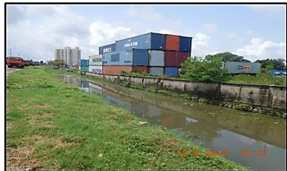
Port Access Road Canal
