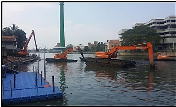
Cleaning of East Beira Lake (Dredging Work)
