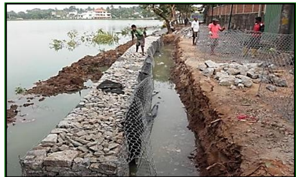
Gabion wall Construction for bank of the lake
