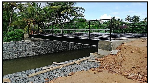
Development at Matara - Stage I
