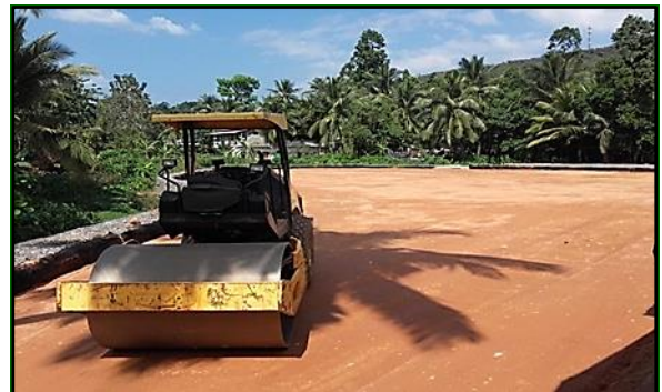
Ground preparation for pola area
