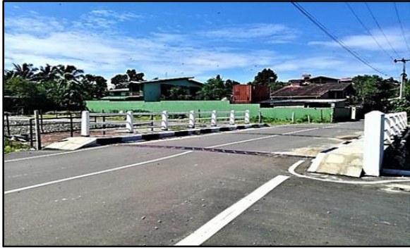
Sooriyamal Mawatha Bridge
