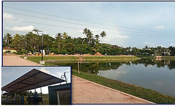
Maintenance work of Walkway in Katubedda
