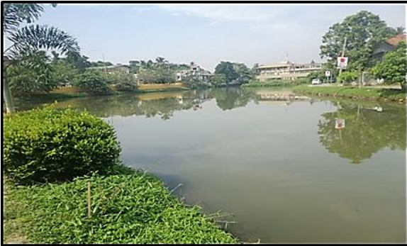
Surface clearing work of Lake at Sudarshanarama Viharaya
