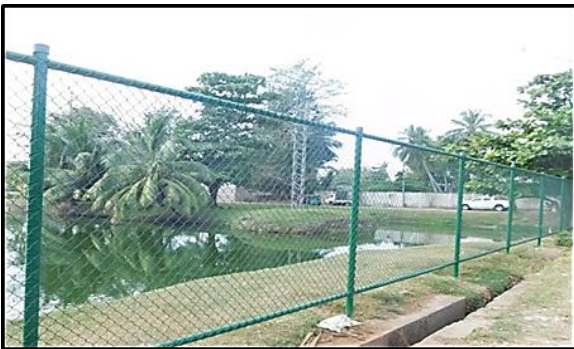
Chain Link fence along the Attidiya Lake II
