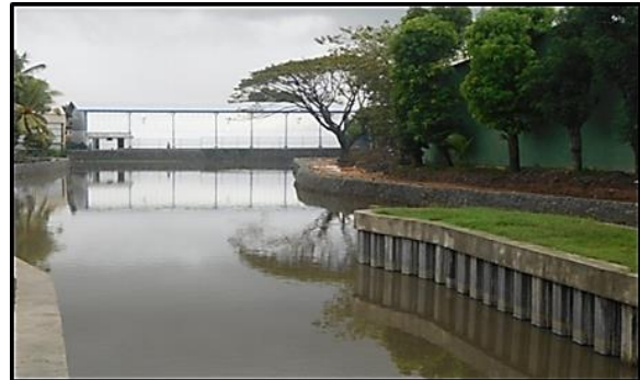
Inflow Canal to the Pump House
