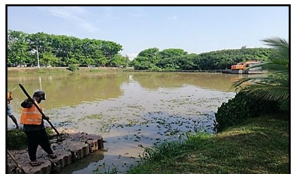
Dredging of Palamthuna Junction Lake
