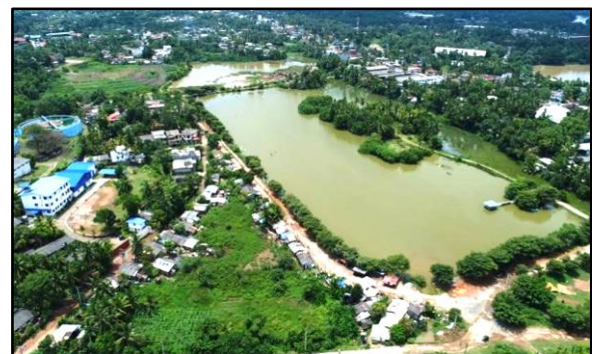
Existing flood situation
