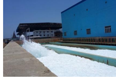
Cooling Inlet & Outlet
