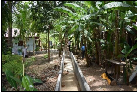
Drainage system to prevent flooding in Galthambarawa in Polonnaruwa
