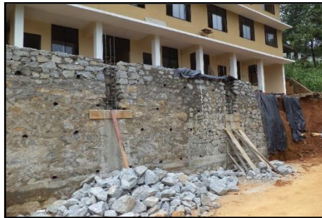
Construction of a safety dam in Nawalapitya Kadireshan Vidyalaya to mitigate landslide risk.
