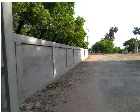
Figure 11 Construction of boundary wall
