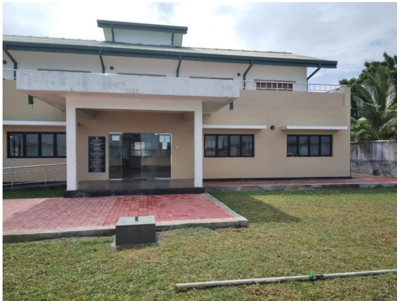
Figure 14 - Administrative Building for the Merchant Shipping Secretariat
