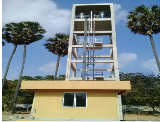
Figure 08 - Elevated water tank and pumping station
