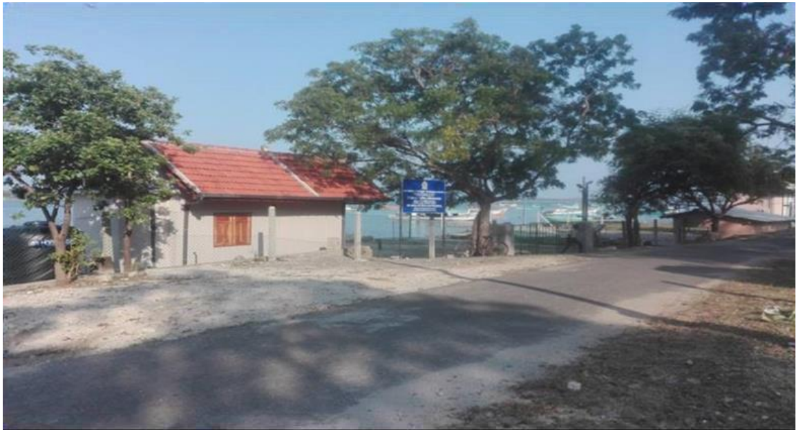
Figure 16- Launchway access and winch house in Kayts
