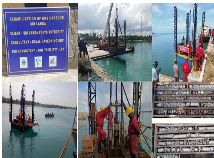
Figure 5- Commencement of Borehole Investigations
