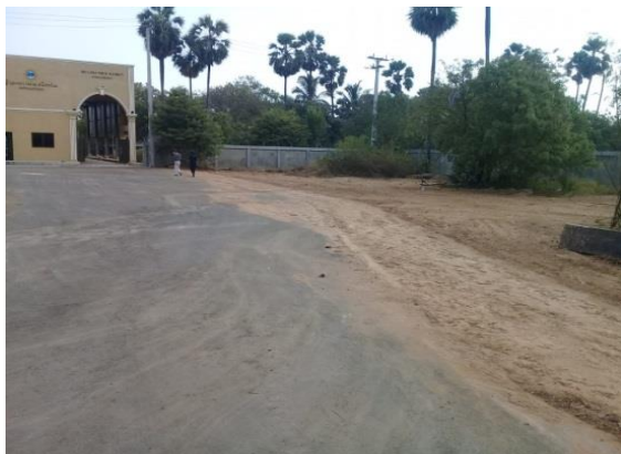
Figure 10- The access path is prepared
