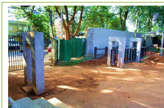
Pic 1.9 – Emergency Gate and Fence
