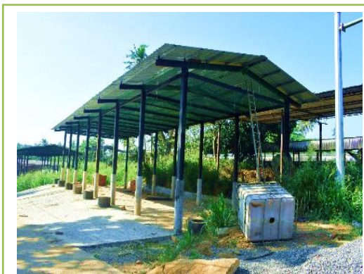
Pic. 1.7 – Construction of new elephant sheds
