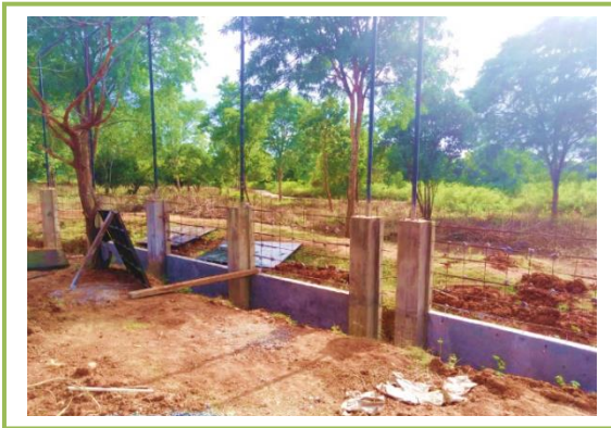
Pic 1.20 – 16' height Chain Link Fence In between Asian Elephant Zone and Cheetah Zone
