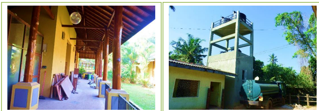
Pic 1.11 - Repairs of the entrance complex and other works
