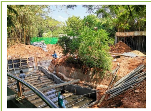
Pic 1.5 - Lion enclosure under construction
