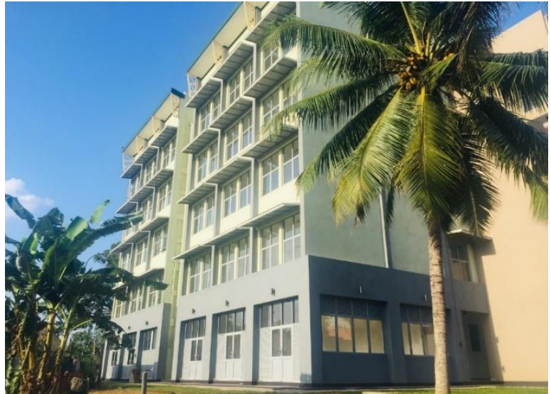
Figure 2: Five Storied Academic Building- Gampaha
