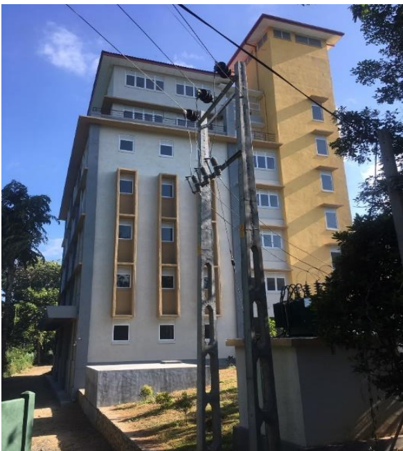
Figure 3: Five Storied Academic Building- Kandy
