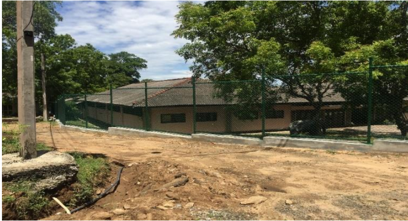
Figure 4: Chain Link Fence- Ampara
