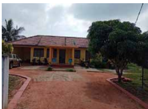
Renovated office quarters of Murungan VS Office
