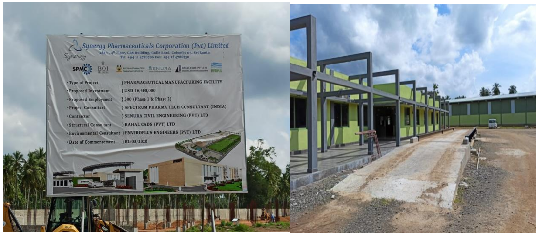
Synergy Pharmaceuticals Corp Pvt. Ltd-Under construction at Bingiriya
