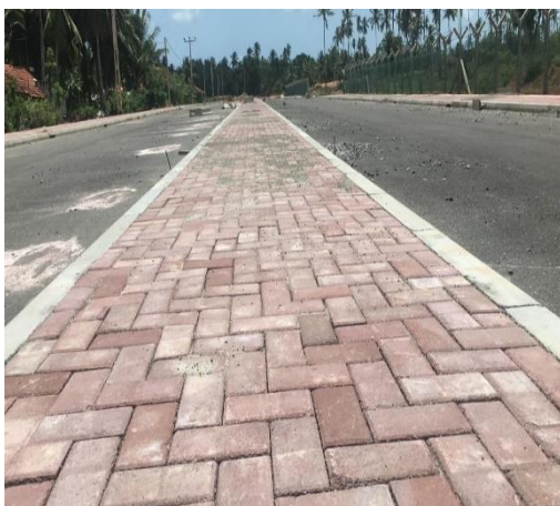
Progress of infrastructure facilities Road Construction Work at Bingiriya
