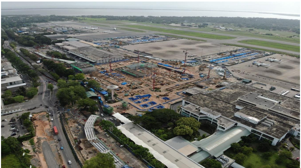
Sky view of the Proposed Bandaranaike International Airport Development Project
