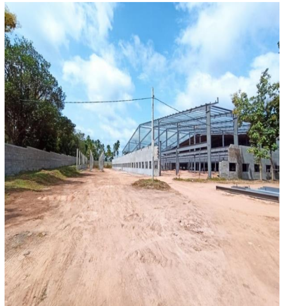
M/s Shanghai Dongxia Industrial & Commerce Co.Ltd.-Under Construction
