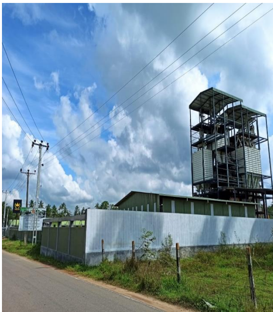
Empire Feed Mill- Under Construction
