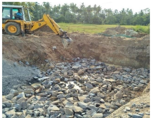
Infrastructure facilities Culvert Construction Work at Bingiriya
