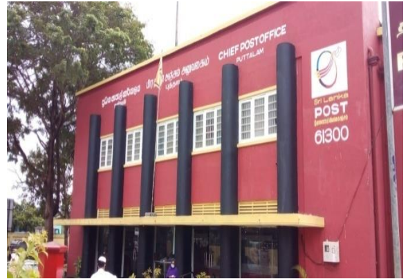
Figure 2.17: Modernization - Post Office, Puttalam
