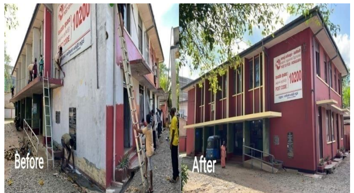
Figure 2.19: Modernization - Post Office, Homagama
