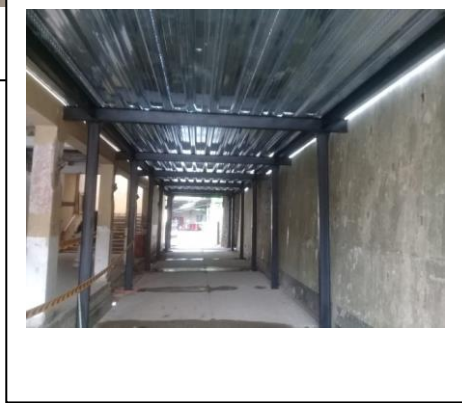
Development works at Nanu Oya Railway station
