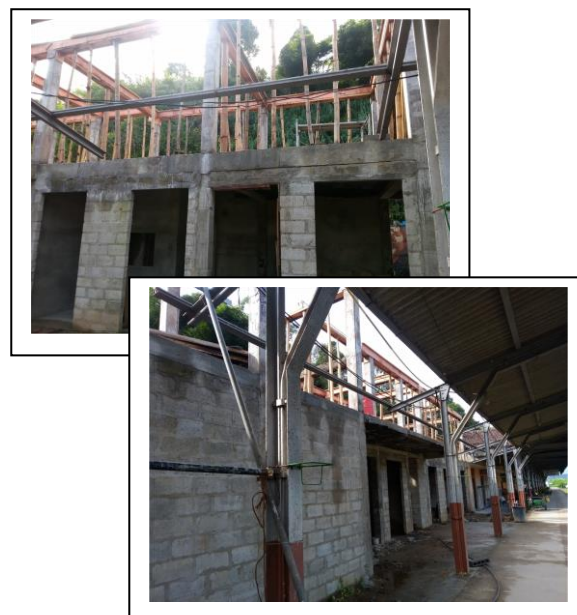
Development works in two story building at Bandarawela Railway station
