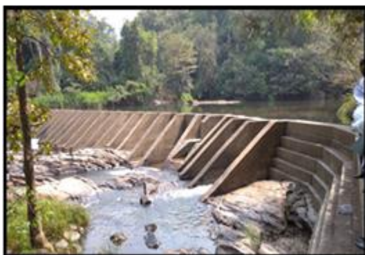
Construction of Water Intake, Wilgamuwa
