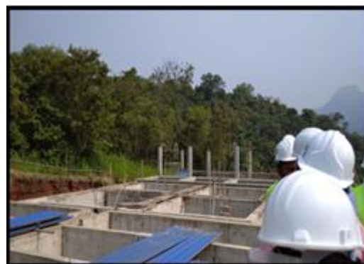
Construction of Water Treatment Plant, Wilgamuwa
