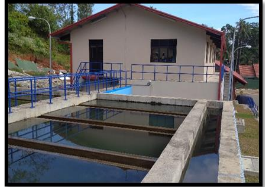
Water Supply and Sanitation Improvement Project, Galigamuwa
