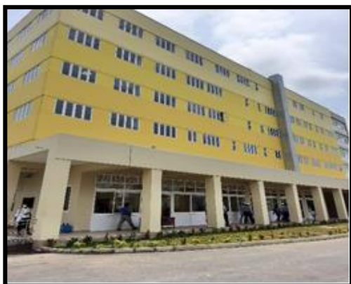
Construction of Helmutkhol Maternity Hospital. Galle
