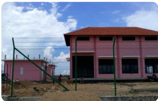
Completed Clear Water Sumps and Pump house
