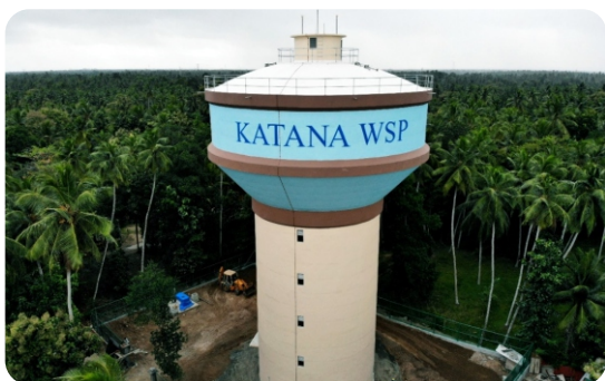
North Tower - Bambukuliya
