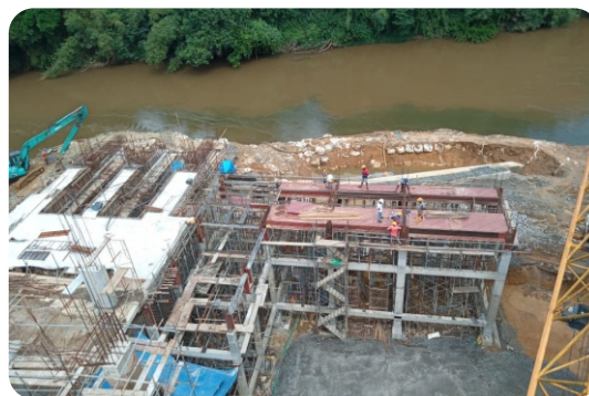
Construction of New Intake at Kolemmodara
