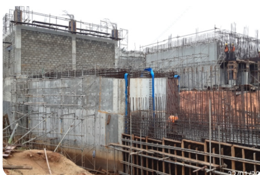
WTP Site - Intake
