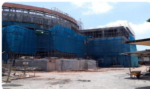
New Training Center and Accommodation Facilities
