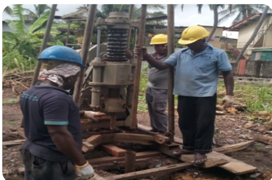
Soil Investigation Work at Pump Station Lands
