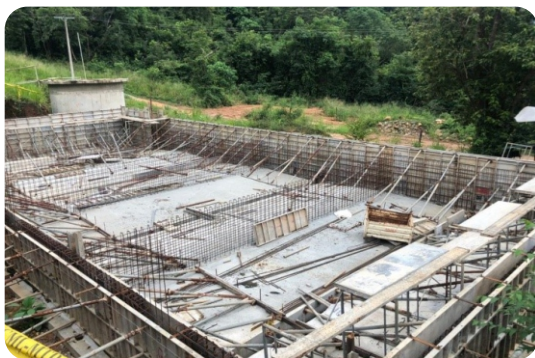
Water Treatment Plant
