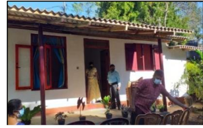
Construction of Child Protection Care House in Thiththapajjala Division.
