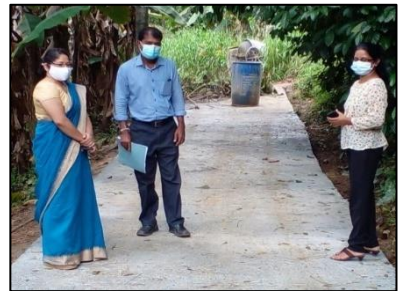
Infrastructure Development Project under “Saubhagya Production Villages” Development of road from Mr. Piyadasa’s house up to Mr. Aththanayake’s House Allocation Rs .500,000.00 Progress Rs.48780.88
