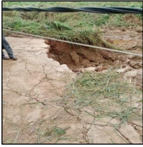
Erosion of Bank of Galagediyawa oya cause to Heavy rain in 13.08.2021
