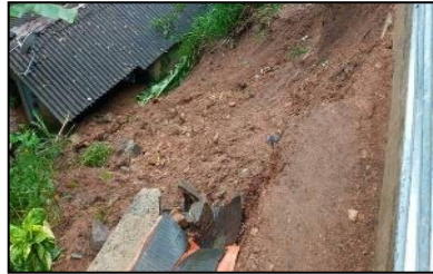
Landslide in Doluwa Nillamba Upper Village due to heavy rains (10.07.2021)
