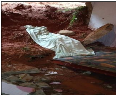
Landslide in meeyanagolla, Ganga Ihala Korale Divisional Secretariat Division
