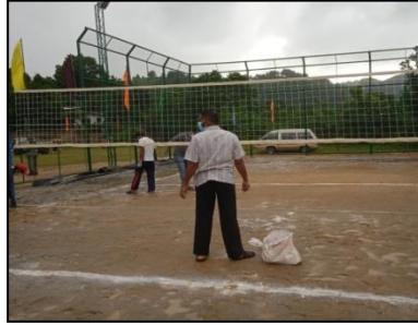
Development of Udispaththuwa mahaweli ground Allocation Rs.1500, 000.00 Progress Rs.1470, 000.00
