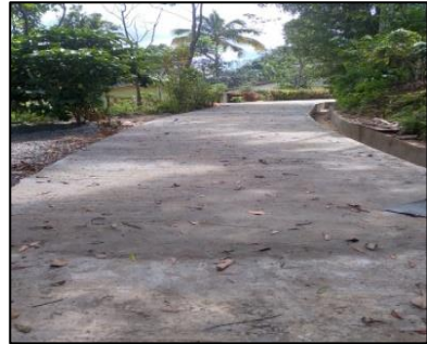
Kataram Colony Road Development Allocation - 4.5 million Financial Progress - 100%
