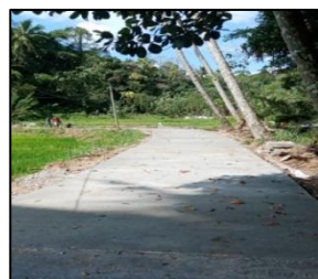
Development of Polgaswewa road of Pallebokalawela with side wall.
