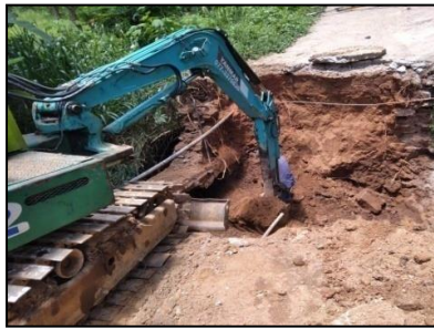
Construction of bridge of Maharawila in Madadumbara divisional secretariat division
