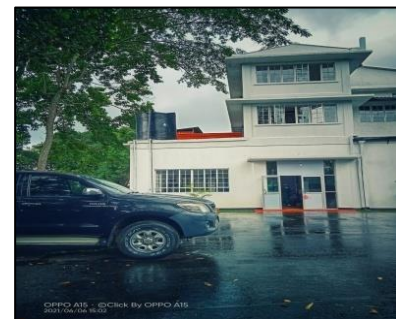
Construction of Covid-19 Hospital in Ganga Ihala Korale Divisional Secretariat Division
