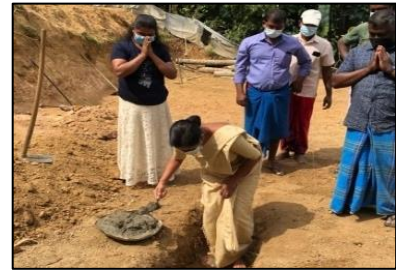
Laying foundation stone for a house to a family who suffer from critical situation of landslide in Pathahewahata Division under patronage of political leaders in division.
