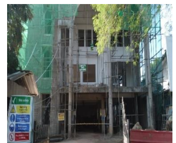
New office building underway.
