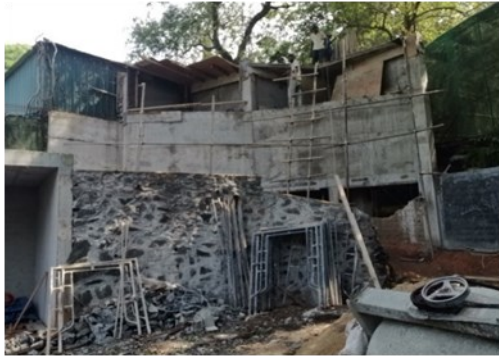
Renovations at the Lion enclosure
