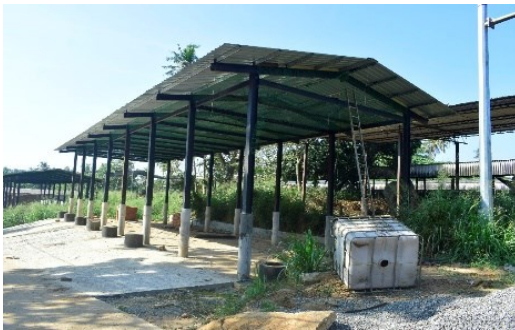
Construction of new elephant sheds
