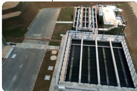
Puttalam Water Treatment Plant
