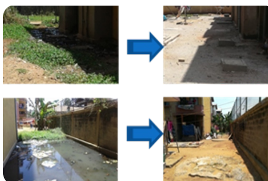
DEWATS for Lunawa Samudra Shakthi HS
