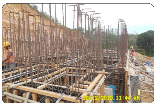
Coagulation & flocculation tanks
