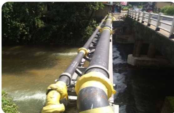
Pipe laying across the Bridge No. 53/3, Avissawella
