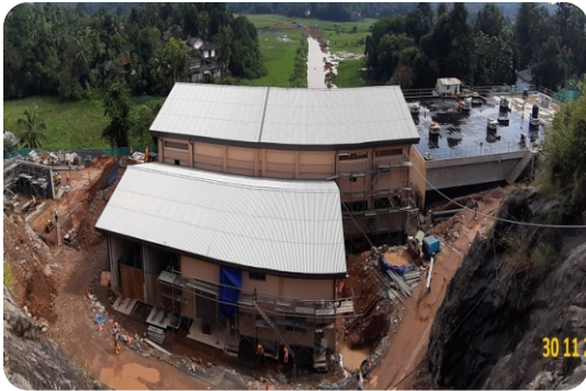
WTP Construction progress
