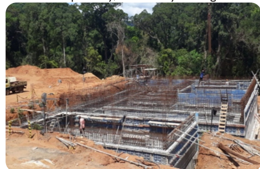
Construction of Clear Water Reservoir at WTP
