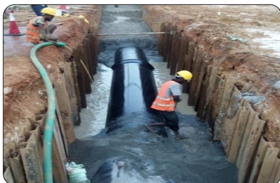
Orugodawatta Pipe Laying
