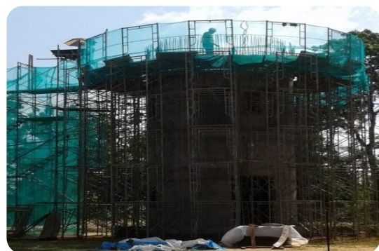
Kotawehera Water Tower
