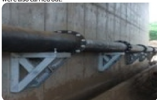
Highway underpass pipe laying at Bandagiriya
