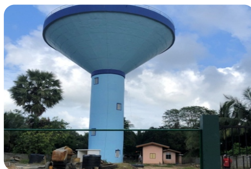
Serunuwara Tower Construction
