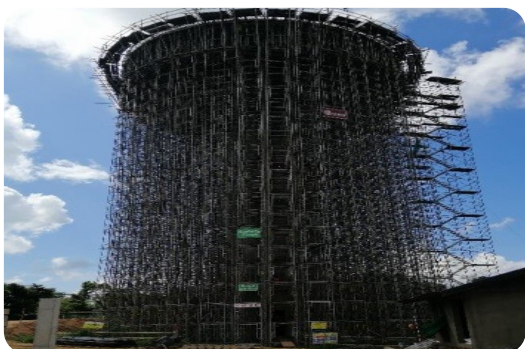
Ethakada Elevated Tower
