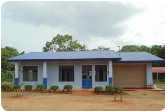
Office Building at New Town tower Premises
