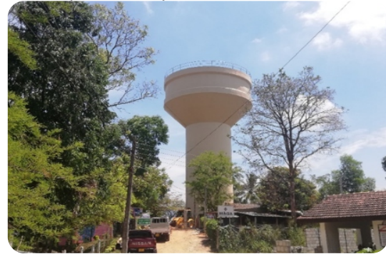
1,000 cu.m capacity water tower at Mawathagama
