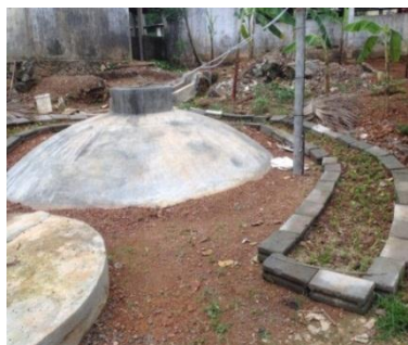
Biogas Digester at Boys Town –Diyagala
