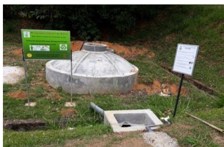
Two biogas digesters constructed for biodegradable waste at CEB village in Kothmale.
