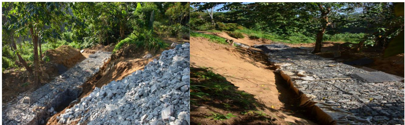
Construction activities of Gabion Wall at Royal botanic Gardens, Peradeniya
