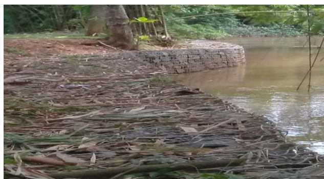
Gabion wall constructed along the Gampaha Botanic Gardens for conservation of the bank of the Attanagallu Oya
