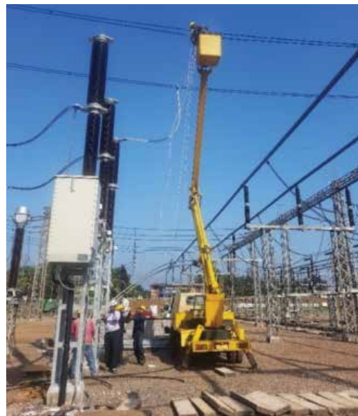
Figure Tr.12: Down dropper replacement work
