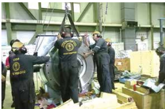
Installing the new TCA66 Turbocharger
