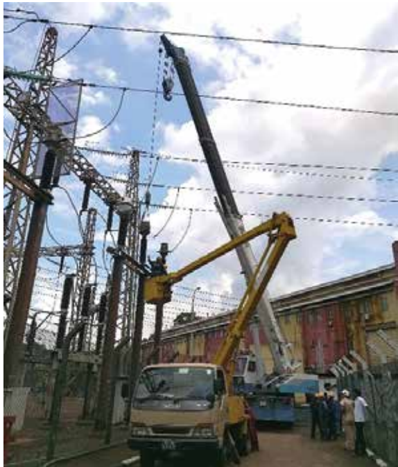
CT Replacement of Switch Yard
