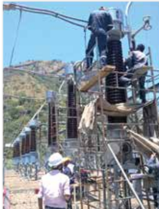
Installation in progress
