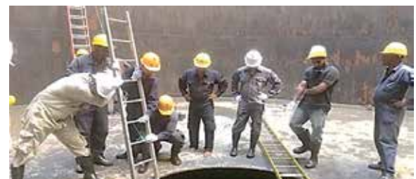
Accessing to Tunnel
