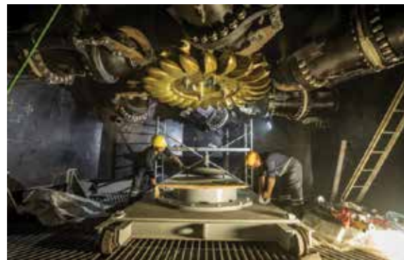
Installation of Turbine (Unit1)
