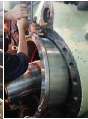
Insertion of Trunnion Bearing
