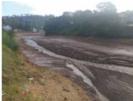
Sedimentation at upstream
