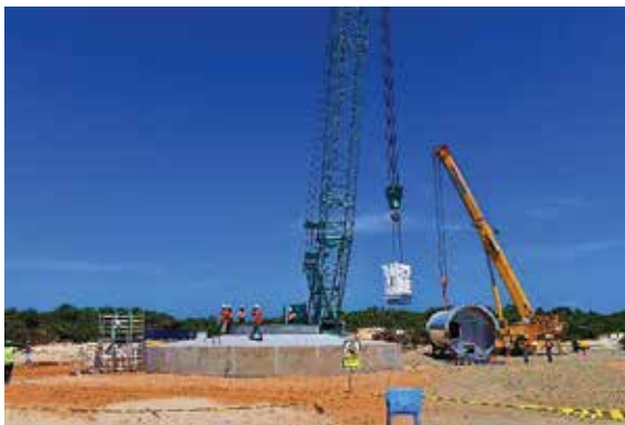
Installation works in progress - MWPP
