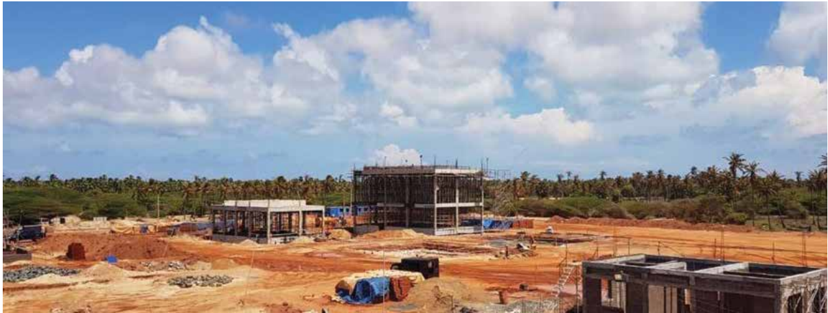
Construction works at Nadukuda GSS 220kV switchyard
