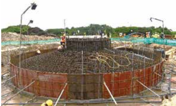
Site works in progress- MWPP
