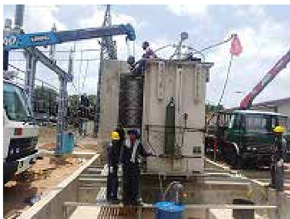
Figure Tr.11: Transformer maintenance work
