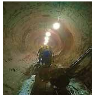
Inside the Tunnel
