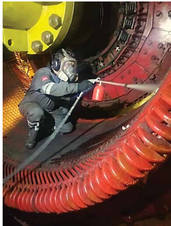
Stator winding cleaning of Generator No.04
