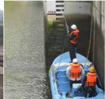
Inspection of Intake Dam Concrete Surface
