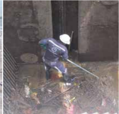
Cleaning the Intake control system
