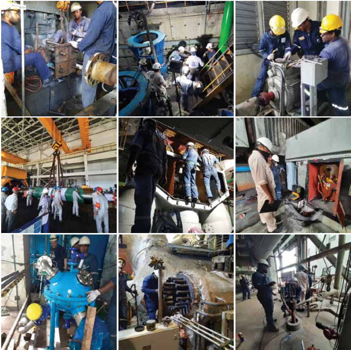
Unit 01 Overhaul- Lakvijaya Power Plant
