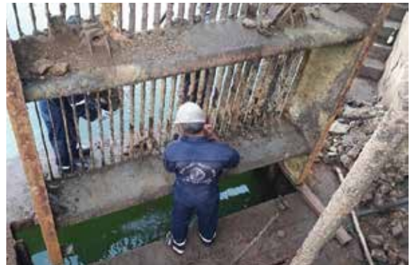
Repairing of trash rack
