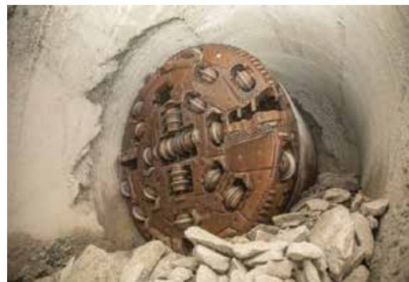
Main Tunnel Breakthrough
