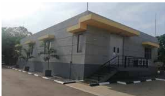
Kelanitissa 33kV GIS substation
