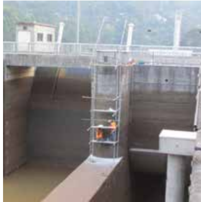
Installation of anchor bolts for the debris
