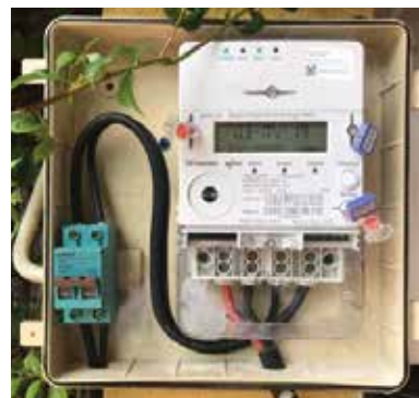
Smart meter installation under pilot project
