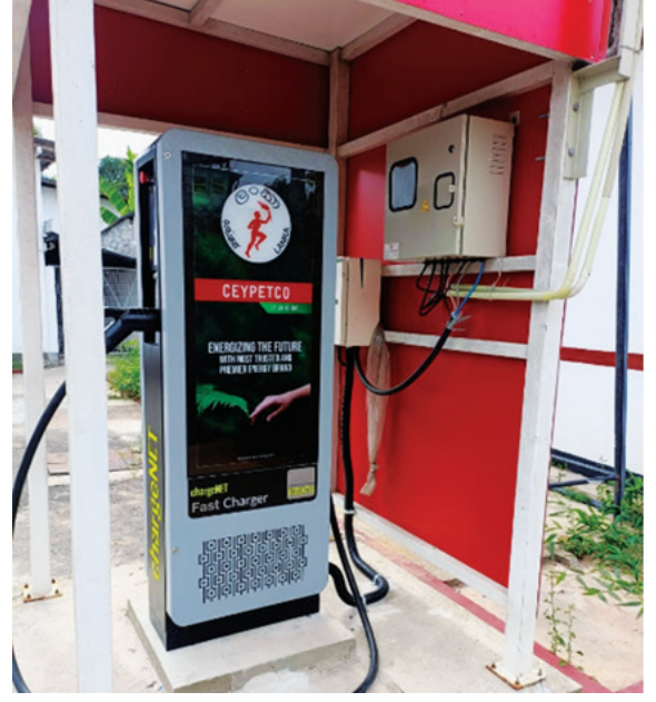
Establishing EV charging stations
