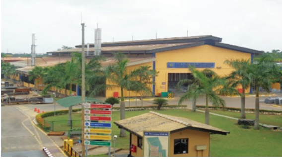
Galvanizing Plant at Sapugaskande
