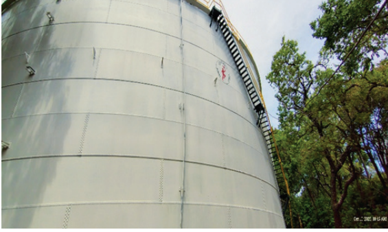
Developing of 24 Trincomalee fuel tanks
