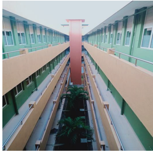
DGH Hambanthota - Isolation Building
